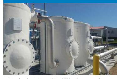
gallon digester tanks, and the 2020 system upgrade provides design features to facilitate installation of a fourth digester. The biogas produced by the anaerobic digestion process is collected, cleaned, and trucked to the Dane County Renewable Natural Gas Processing and Offloading Station. From here the RNG is injected into the interstate transmission pipeline so it can be used as renewable fuel, powering fleets of RNG vehicles across the United States.
