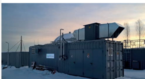
Biogas: 100 Nm 3 /hr Biomethane: 55 Nm 3 /hr
