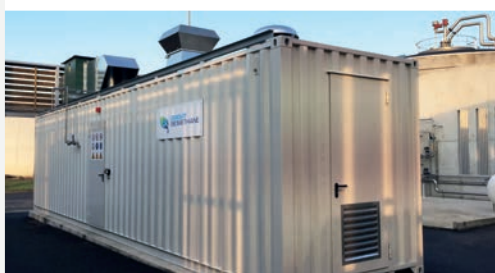
Biogas: 190 Nm 3 /hr Biomethane: 107 Nm 3 /hr
