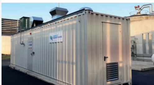
Biogas: 190 Nm 3 /hr Biomethane: 107 Nm 3 /hr
